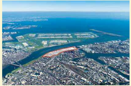
KING SKYFRONT, an international innovation hub located in the Tonomachi International Strategic Zone, continues to attract more companies and R&D institutions.
