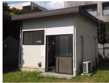
A measuring station
