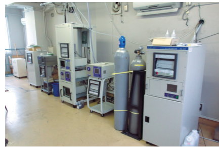
Air-measurement equipment in a measuring station
