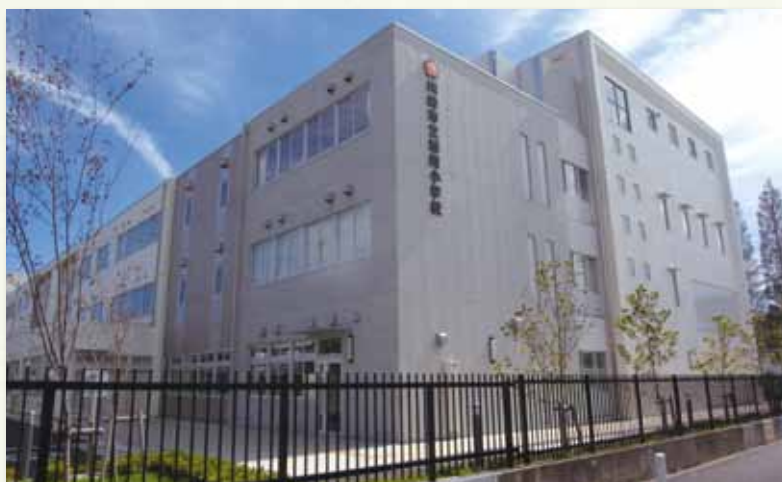
各公立学校の状況に応じた環境配慮技術導入型の改築・改修工事を実施 Implementing the reconstruction and refurbishment work using environmentally-friendly technology, according to the conditions of each public school building.
