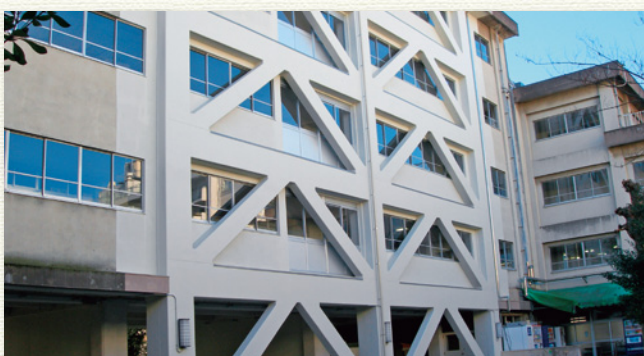
公共建築物耐震化推進事業 Earthquake-Resistant Retrofitting of Public Buildings
