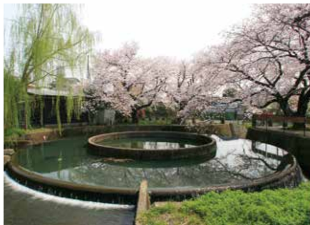
先人の知恵が詰まった国登録有形文化財「二ヶ領用水久地円筒分水」 "Nikaryo Aqueduct Kuji Ento Bunsui", a cylindrical water division system that is one of the national registered tangible cultural assets
