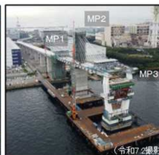
②主橋梁部MP1～MP3
