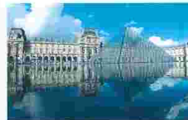
Photocatalysis acts as an antifouling and antifogging effect simply by the irradiation of light. It has also been used in the glass covering the pyramid-shaped entrance of the Louvre Museum. The glass maintains its transparent beauty by decomposing dirt.
