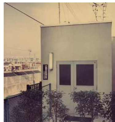
Hirase River Water Quality Monitoring Station
