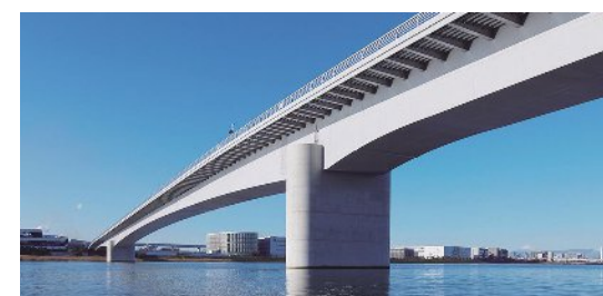
Tamagawa Sky Bridge
