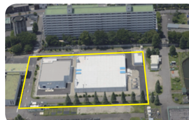
Hirama Distribution Station Regulates a distributed amount and a distributed pressure to the coastal areas having many factories which consume the water resources for industrial use. In accordance with our restructuring plans we renovated the regulating reservoirs and other facilities, and they were put into full operation from FY2016.
