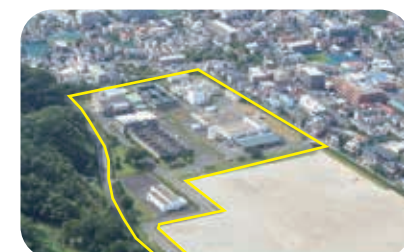
Nagasawa Purification Plant Started passing water in June 1954. The original water is river water from the Sagami River, the treatment method is coagulation sedimentation process, and the water supply capacity is 235,000 m 3 /day. A regulating reservoir and other facilities were constructed under the Restructuring Plan.
