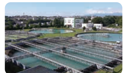
Nagasawa Purification Plant Regulating Reservoir Constructed under the Restructuring Plan and put into full operation starting from FY2013. Reservoir and other facilities were constructed under the Restructuring Plan.
