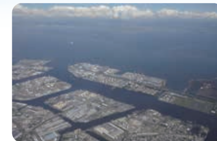
The water resources for industrial use are more economical than tap water and used for cooling, cleaning, etc. at the petrochemical factories, ironworks, etc. in the Keihin Industrial Zone in the coastal areas. (Photo: Coastal area, adjacent to Higashiogishima)
