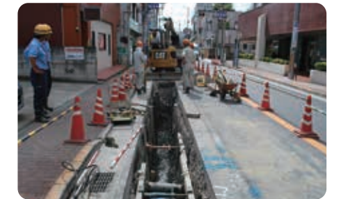
Earthquake-proofing Water pipes
