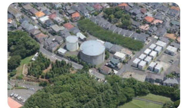
Chiyogaoka Elevated Distribution Reservoir
