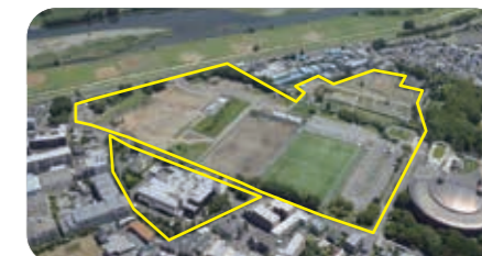
Todoroki Wastewater Treatment Center
