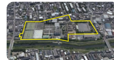
Kase Wastewater Treatment Center
