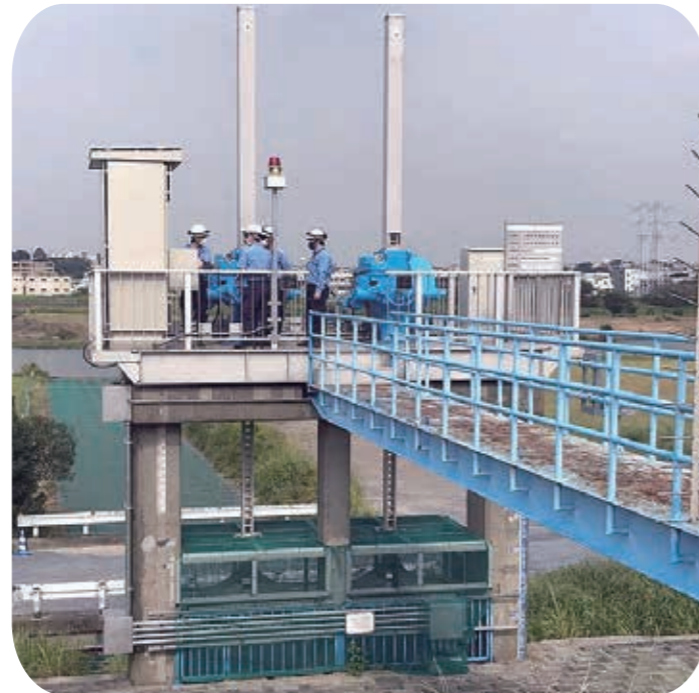
Operation training of drainage flume gate
