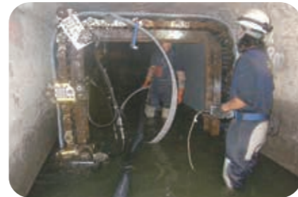
Earthquake-proofing important Water Pipes through Reorganization Measures
