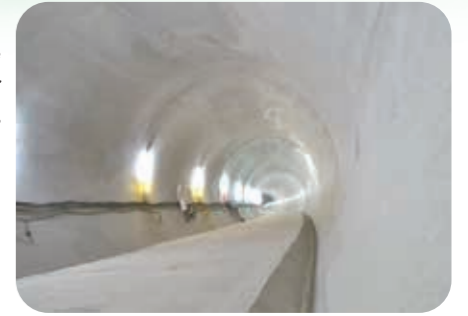
Daishigawara Storage Pipe (Operations started in March 2019)
