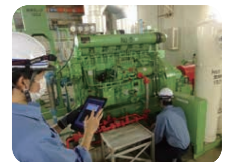
Inspection status of equipment using tablets
