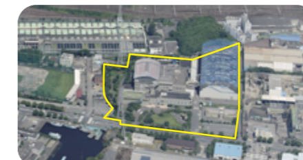
Iriezaki Sludge Treatment Center
