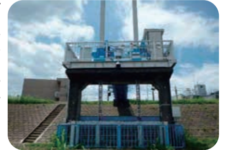
Electrification of drainage gutter pipe gates (started operation in July 2020)
