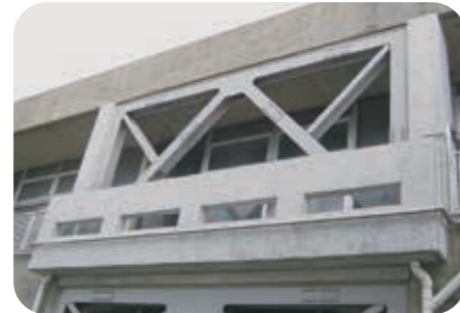
Earthquake proofing Buildings under Construction (by using braces etc.)
