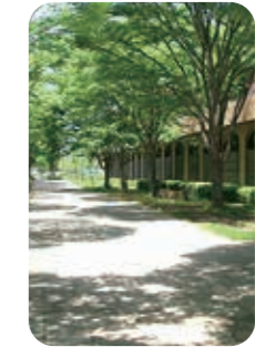
Asao Wastewater Treatment Center
