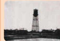
Tode Purification Plant
