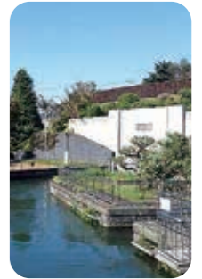
Nagasawa Purification Plant
