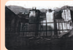
Shiroyama Dam under Construction
