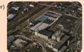
Kase Sewage Treatment Plant
