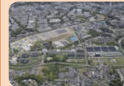
Nagasawa Purification Plant
