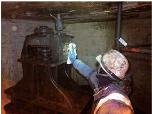
仕切弁保守点検
