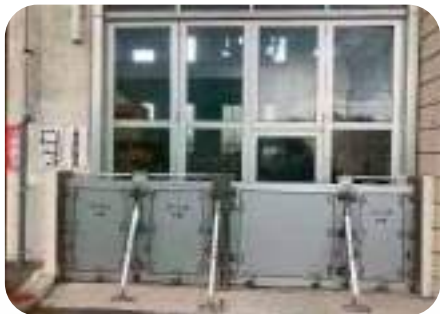
Waterproofing of facilities (watertight panels)
