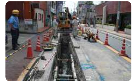
Earthquake-proofing Water pipes
