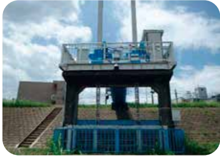
Electrification of drainage gutter pipe gates (started operation in July 2020)
