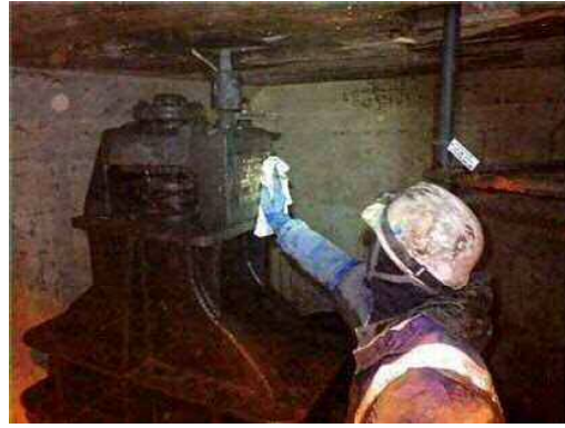
仕切弁保守点検
