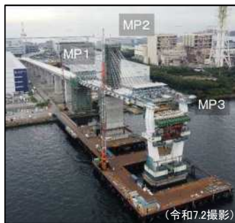
②主橋梁部MP1～MP3
