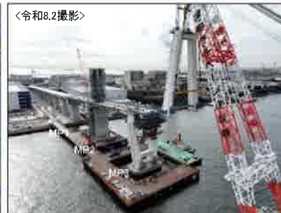
②主橋梁部MP1～MP3
